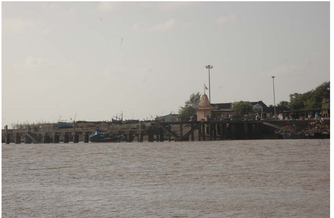
NANI-DAMAN NEW JETTY
