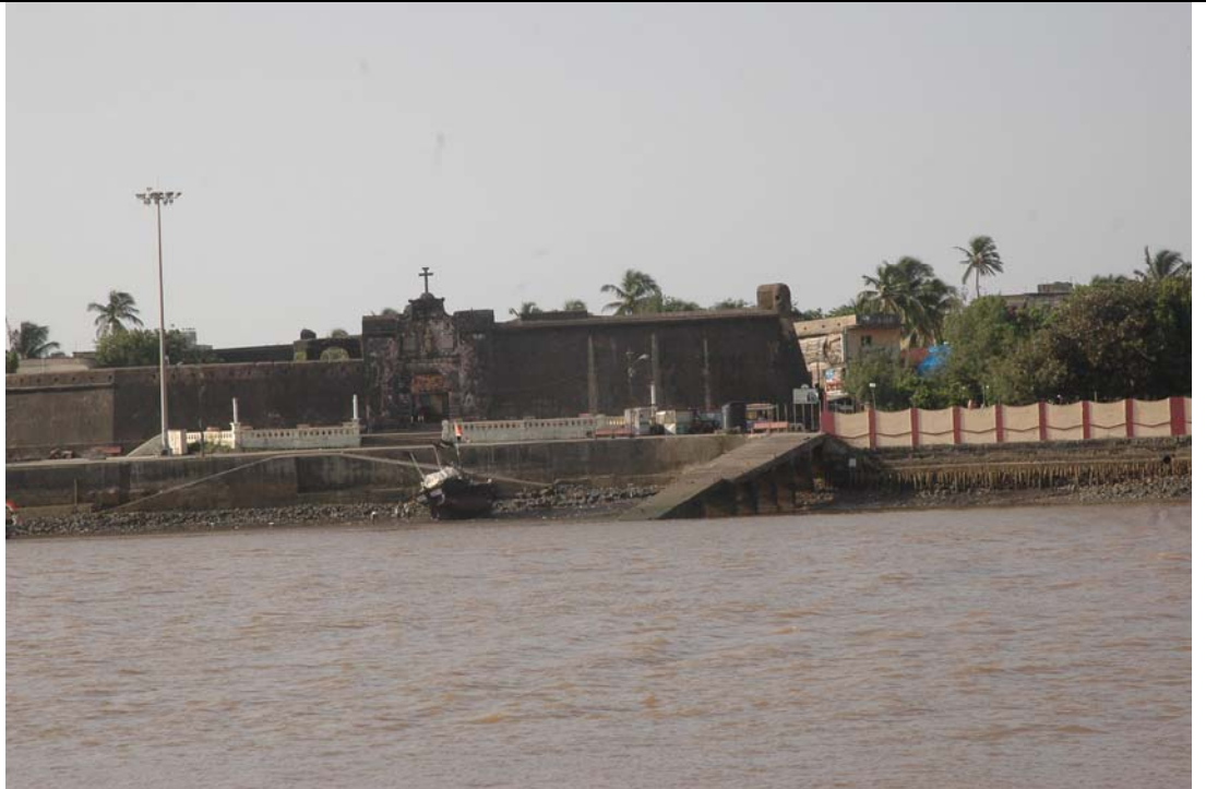
NANI-DAMAN OLD JETTY
