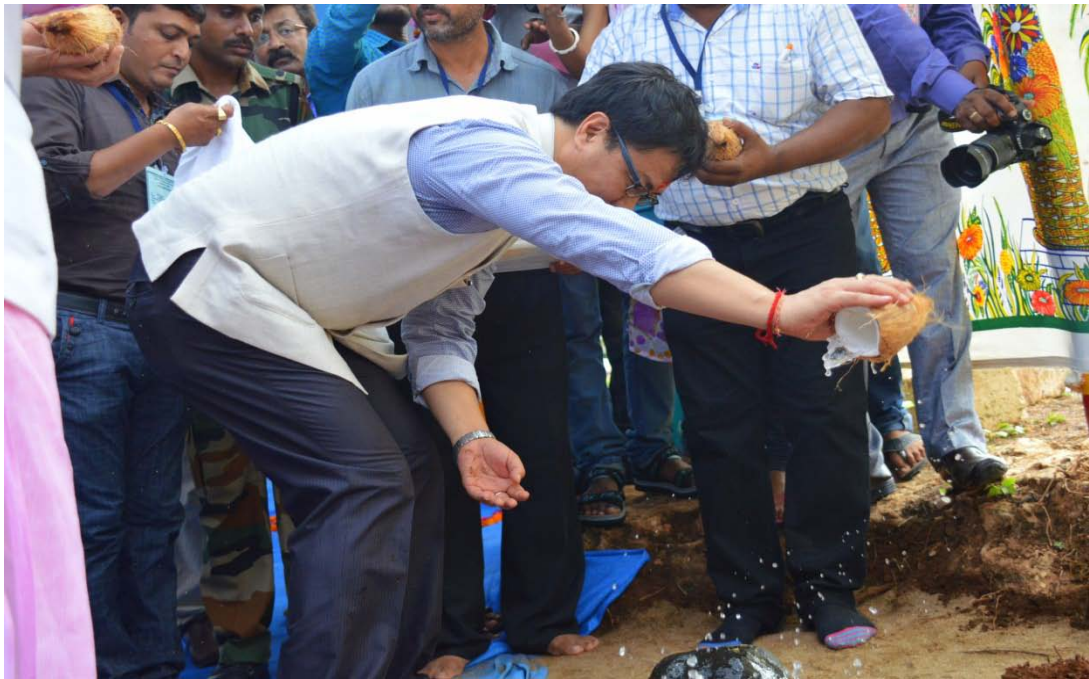
Hon'ble Minister inaugurating Laying Foundation Stone of Tad Bridge at Tad Creek at Diu
